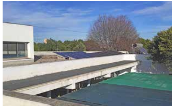
Installation of photovoltaic panels at CEIP Sanchís Almiñano in Alaquás (Valencia).
